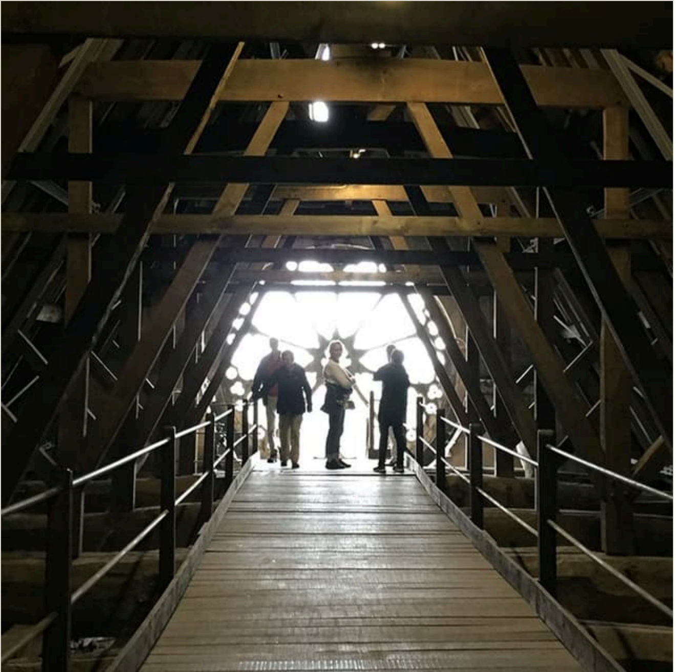
A roof tour, up among the Minster's medieval roof timbers.
